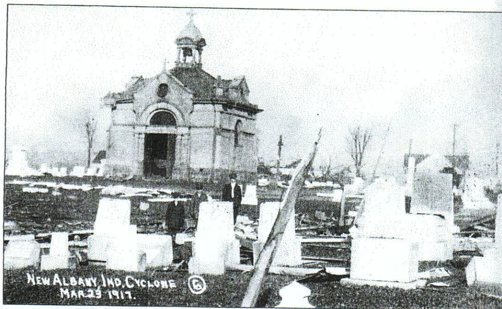
ST. MARY'S CEMETERY. Even marble and stone were prone to damage from the tornado. This image of St. Mary's Cemetery on Charlestown Road shows several stones uprooted or damaged. The chapel in the center is no longer standing.
